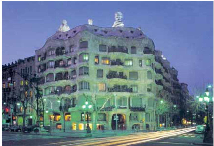
Milà House: Pere Milà had seen the Batlló house and was enthralled by its beauty, so he asked Gaudí to construct a large building of rental flats on his newly acquired land. Its façade, made of stone, gave the house the contemptuous nickname of La Pedrera (the stone quarry) since stones needed were cut in front of the building, occupying the street. (Not a very nice view...). The roof is peculiar, because it is replete with strangely shaped chimneys and ventilators and from it you can make out all the sights of Barcelona.
